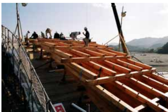
Photo 21: Bridge Girder Assembled on Site
