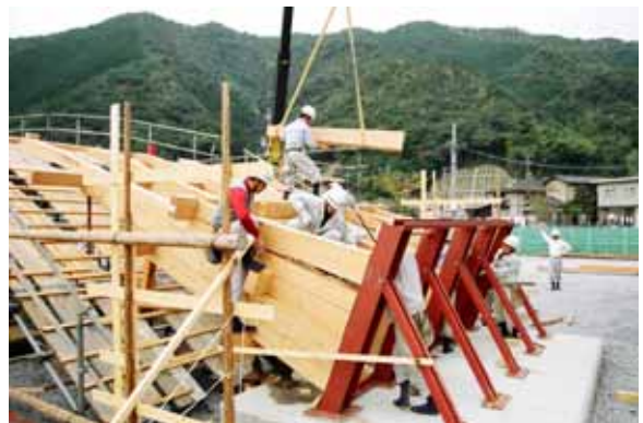
Photo 17: Bridge Girder Assembled on Land
