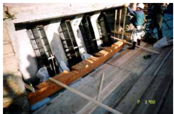
Photo 18: Installed Crossbeams
