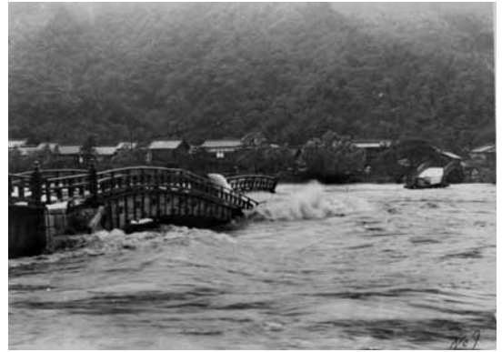
Photo 3: An arch being washed away following the collapse of the fourth pier, due to the erosion of its stone footing
