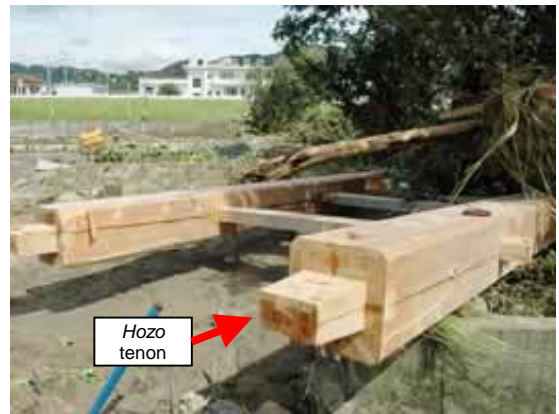
Photo 9: Tapered hozo tenon, a design to enhance the ease of disjoining
