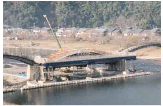
Photo 24: Alternative bridge installed during the first phase of the project
