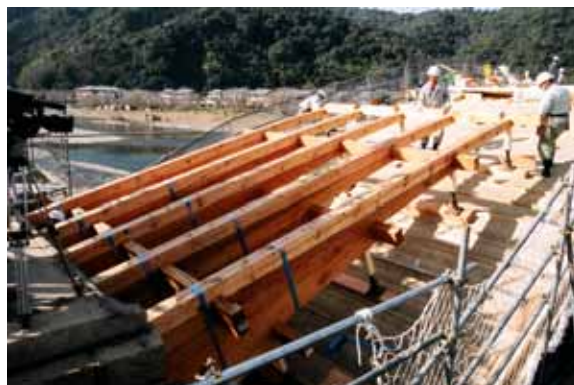
Photo 20: 1st through 4th Girder Members Fixed to Iron Shoe
