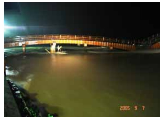
Photo 6: The flood of September 2005
