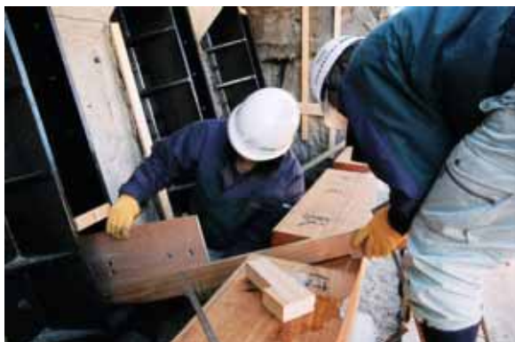
Photo 19: Angle Adjustment of 1st Girder Beam
