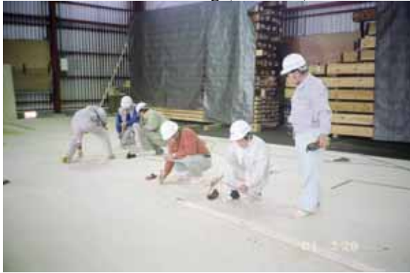
Photo 13: Girder Members Are Drawn
