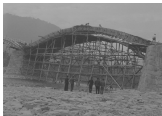
Photo 23: Rebuilding the Bridge during the Showa Period (1926 - 1989) (for reference)
