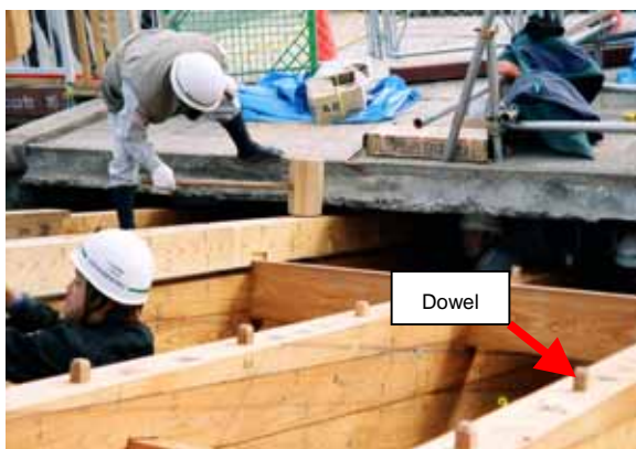
Photo 11: Installed Dowels
