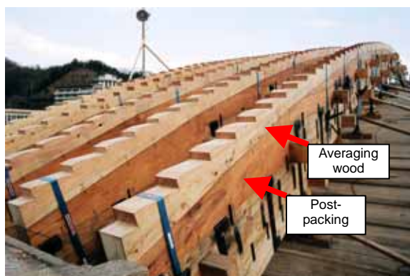
Photo 22: Post-Packing and Averaging Wood Members Installed on Girder Assembly
