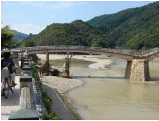
Photo 7: The first span after losing two piers in the flood of 2005
