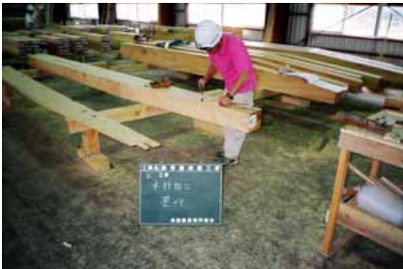
Photo 16: Marking on Timbers
