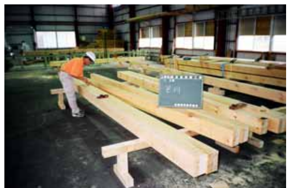
Photo 10: Marking on timbers
